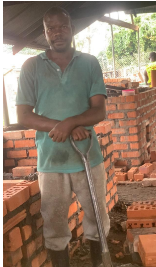
Mr Kato Wilson labouring at the kitchen refurbishment
